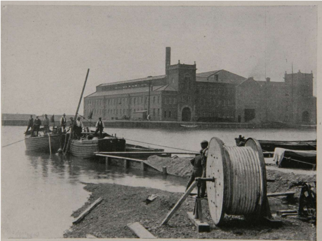
LAYING TRUNK CABLES TO THE NEW POWER STATION.
